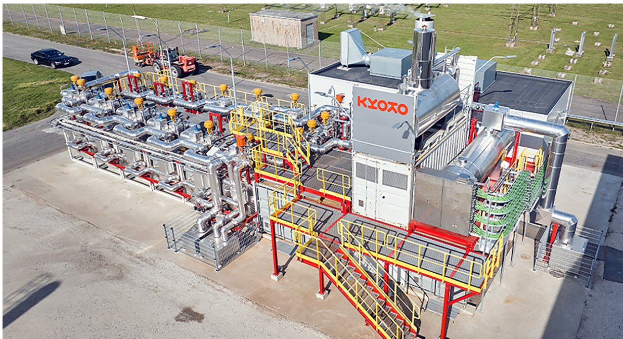
Fig. 3: Heatcube at Norbis Park has replaced coal for district heating in Aalborg, Denmark. It is charged with 5MW and has a storage capacity of 18 MWh. This Heatcube reduces emissions up to 2000 tonnes of CO 2 per year.
